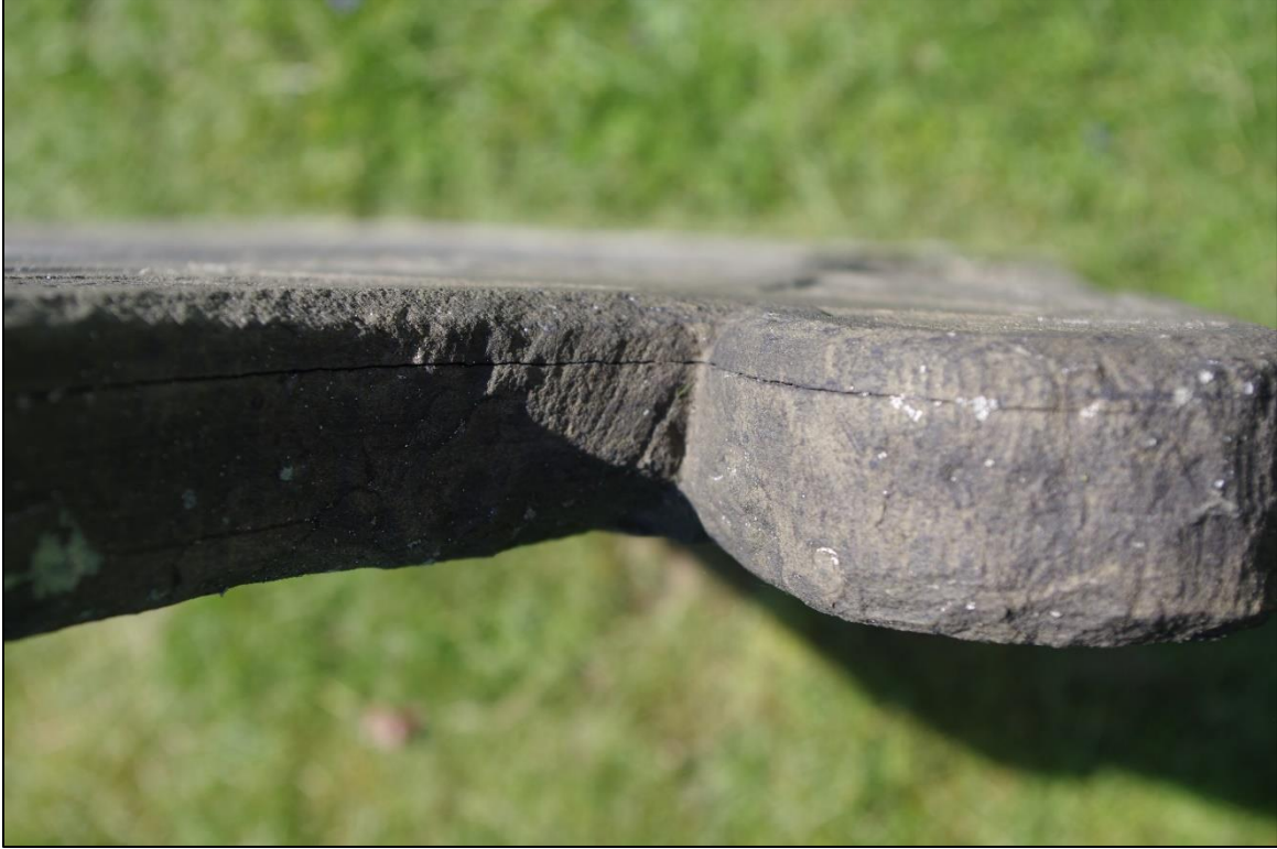
Photo 3. Close-up of Mary Fitch tombstone showing delamination
