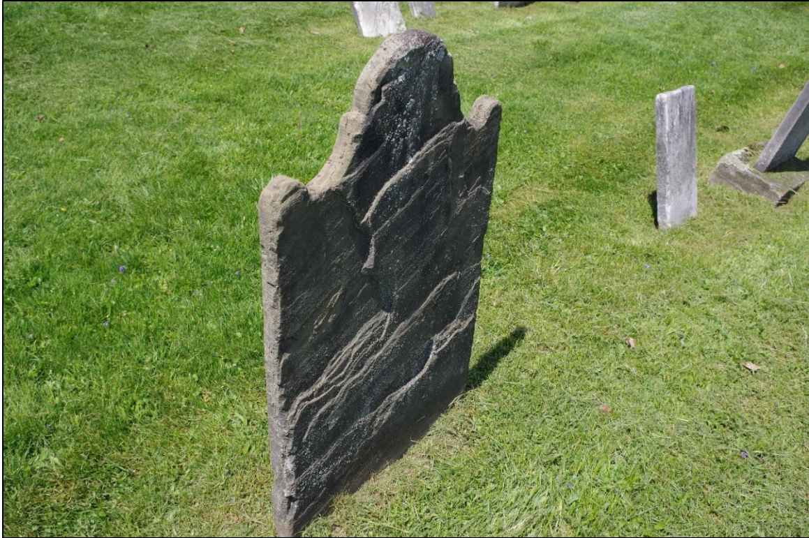
Photo 4. Severely delaminated tombstone with the inscription lost. From context, the stone is that of Susannah (DuBois) Seymour.
