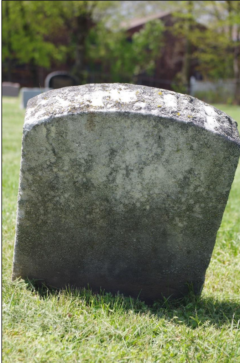
Photo 8. Tombstone, probably of Henry Garnochan, Jr., leaning forward with staining and lichens. Cleaning and straightening may make the stone more readable.
