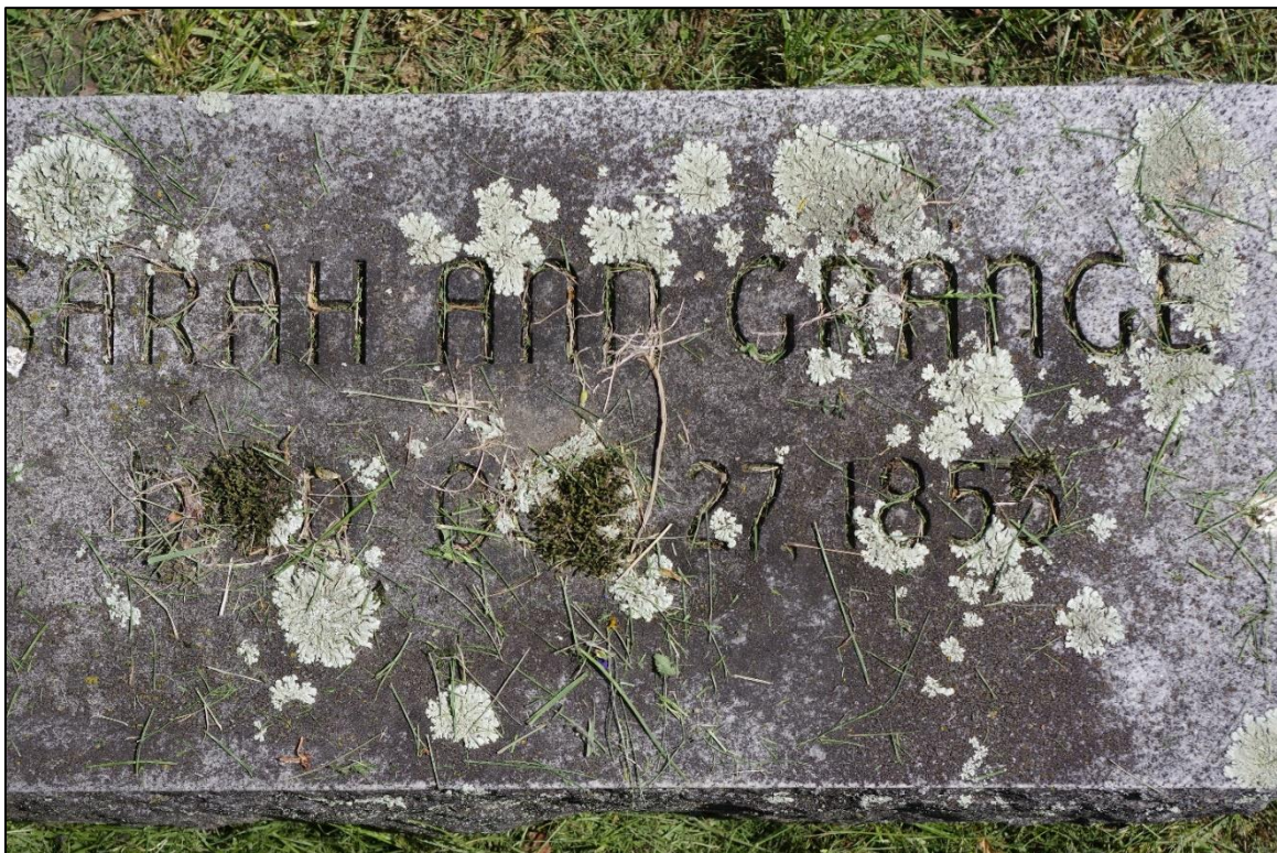
Photo 7. Granite tombstone of Sarah Ann Grange, showing staining, moss, and lichen growth.
