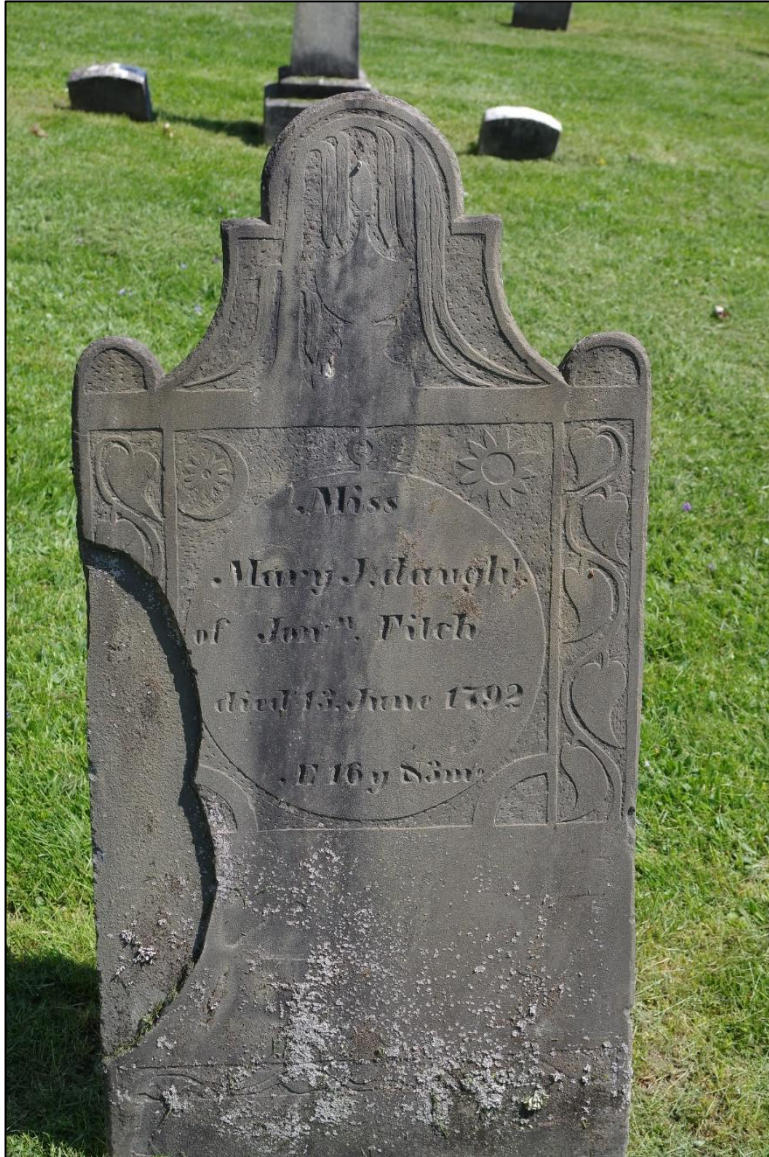
Photo 2. Tombstone of Mary Fitch showing partial delamination with part of the face spalled off.
